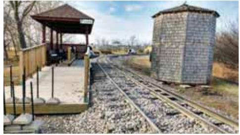
This is a major project - levelling, laying new ties, correcting angles, replacing rail, pounding spikes and putting down truckload after truckload of gravel. WDM Chief Engineer Tim Pomeroy brought in an experienced railway inspector once the work was completed.
