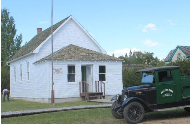
1. List the materials that were used to build this building. Where would local builders get these materials? Wood siding, shingles and walls. Stone foundation. The foundation materials may have been found locally. Wood may have been found locally from sawmills in northern Saskatchewan. If local wood wasn't available, it may have been shipped by rail from larger cities. Windows were likely purchased from a local hardware store or shipped from a
