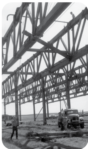
This photo shows the early stages of hangar reassembly in North Battleford
